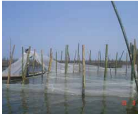
Fig 2. Cage installation in the lagoon
