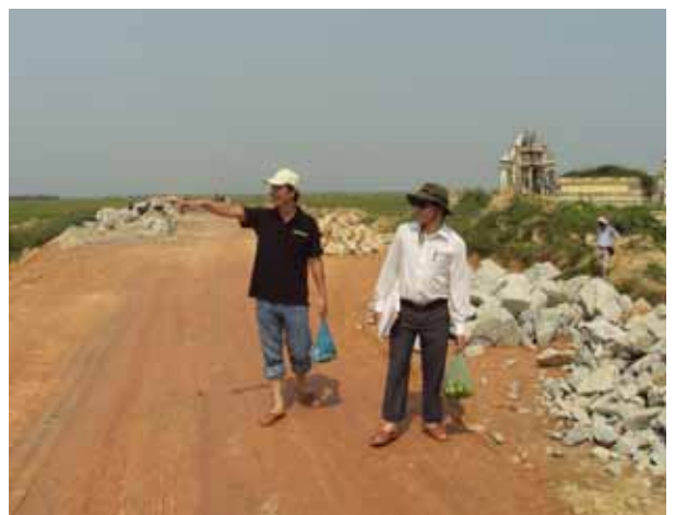
The road constructs nearby Rucha
